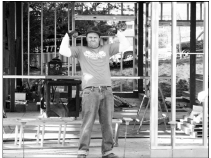
Building the Gym, 2007 (Photo by Traver Normandi)
