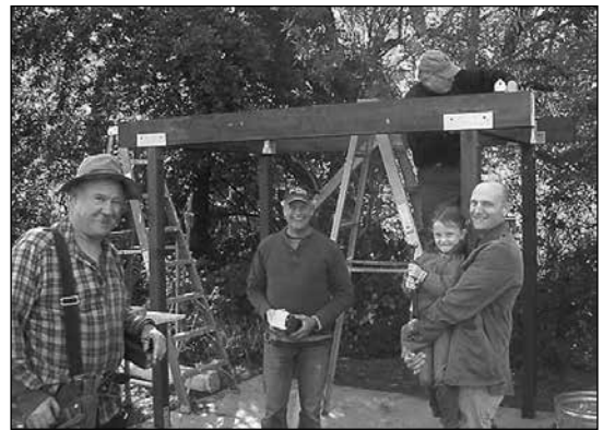
SGV Lions building the Forest Knolls bus shelter (Photo from website)
