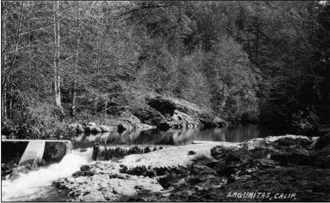
Small dam on creek, Lagunitas (From the Collection of Newall Snyder)
